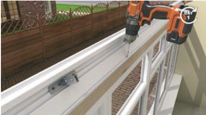
Timber packer and structural ringbeam are sealed and secured to the top of the window frames.
